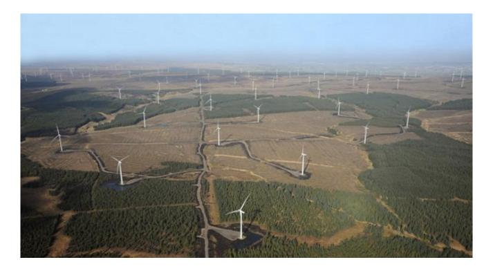
**Description:** 140 turbines; covers 55 km<sup>2</sup>; *peak* capacity of 322 MW  $\Rightarrow$  6 W/m<sup>2</sup> *peak*. Average amount of power produced is small because turbines do not run at peak output all the time. The ratio of average power to peak power is the load factor. Typical value for a good site with modern turbines: 30%  $\Rightarrow$  power production per unit of land for the Whitelee wind farm is  $\simeq 2 \text{ W/m}^2$ .
