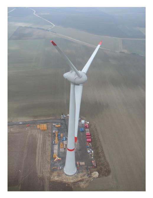
The Enercon E-126 is the largest wind turbine built to date. Technical specificities: bub height of 135 m; rotor diameter of 126 m; can generate up to 7.58 MW of power (or  $\frac{7.58 \times 10^6 \times 24}{1000} = 181,920$ kWh/d).
