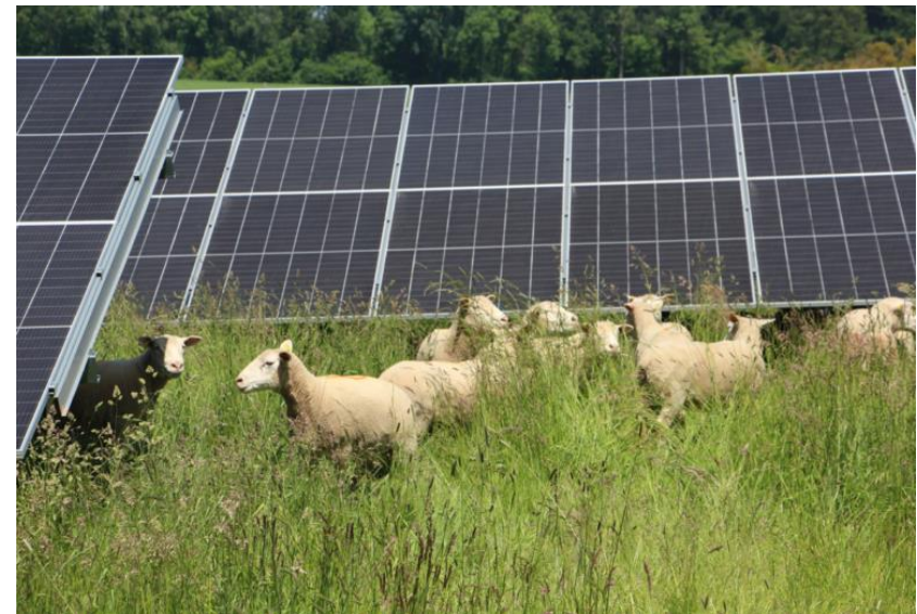
Figure 15: EtherEnergy agri-PV project – Namur.
